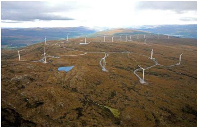
The Millennium Wind Farm initially consisted of 16 x 2.5MW Nordex turbines and associated infrastructure, with an expected life of approximately 25 years. Each turbine is around 115m high from its base to the highest point of its blade.
